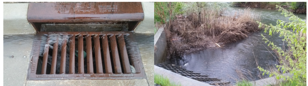
Storm water flows through storm drains directly to local creeks and rivers with NO TREATMENT.
