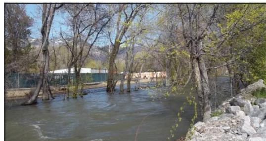
Although the project is not yet complete, the efforts of the contractor to protect the newly shaped stream banks and flood plains with erosion control measures limited effects of the long duration of runoff. The damage that did occur was limited to minor repairs.
